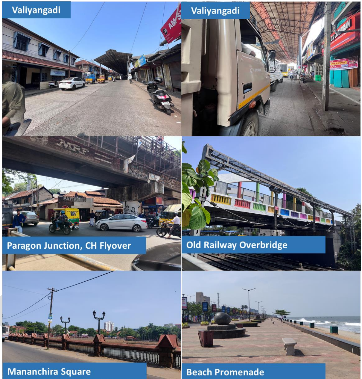
Figure 8-62 Existing Site Situation
