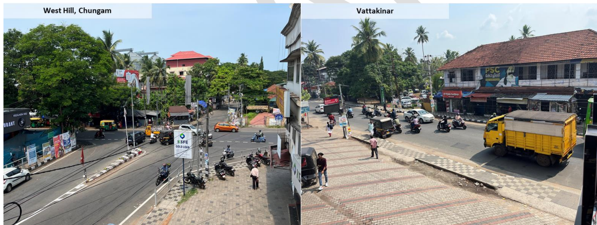
Figure 2-35 Existing Improved Safety Measure for Pedestrian
